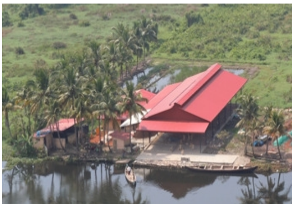
Fig. 1. Aerial View of the AIMS Composting Facility
