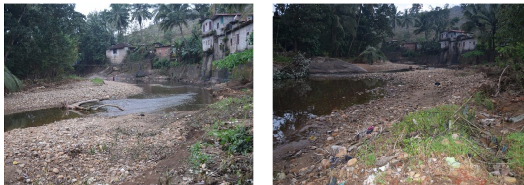
Fig. 9. Theekoy headwaters after the landslide and first flood wave
